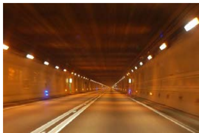
Figure 6. An inside view of the Fréjus tunnel.
